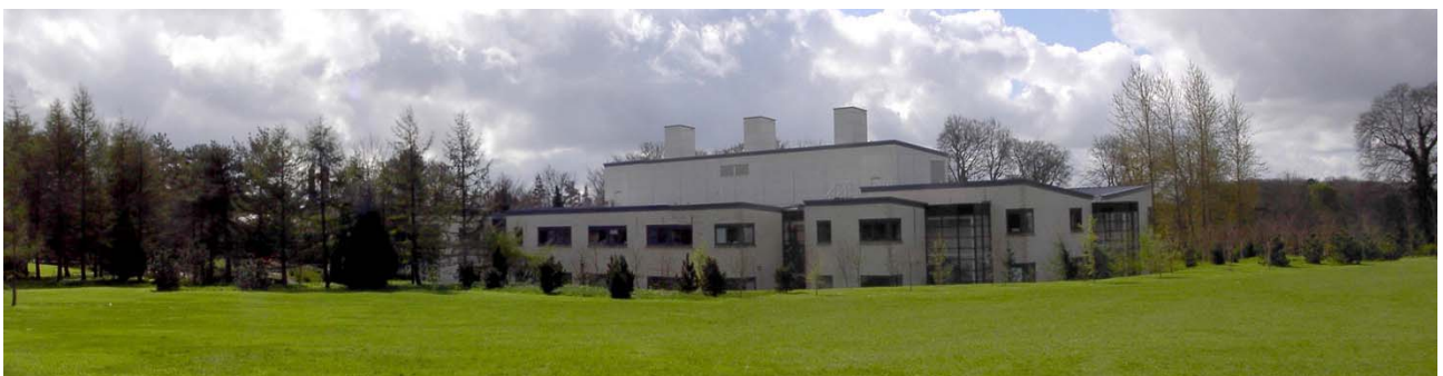
Completed School of Chemistry and associated landscape works
